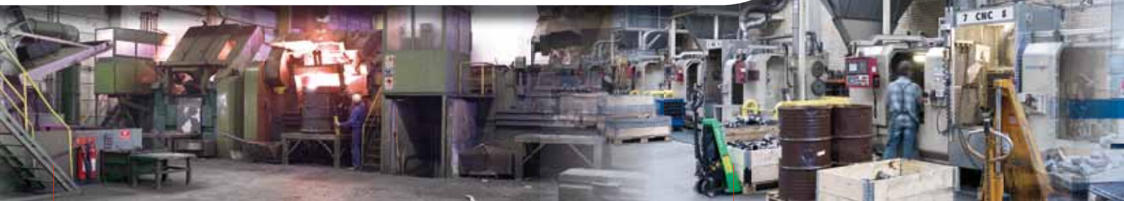
Melting in electric medium-frequency furnaces.
